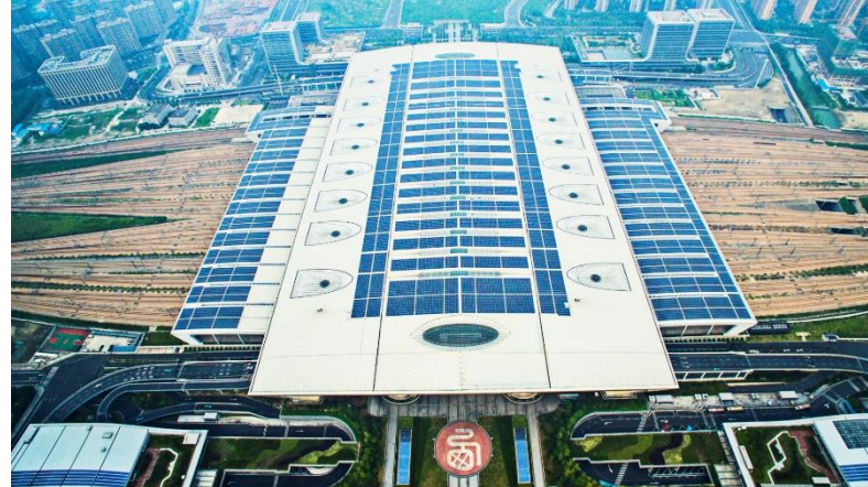
Roof Photovoltaic Power Station of Hangzhou East Railway Station 10MW | Hangzhou, Zhejiang Province, China
