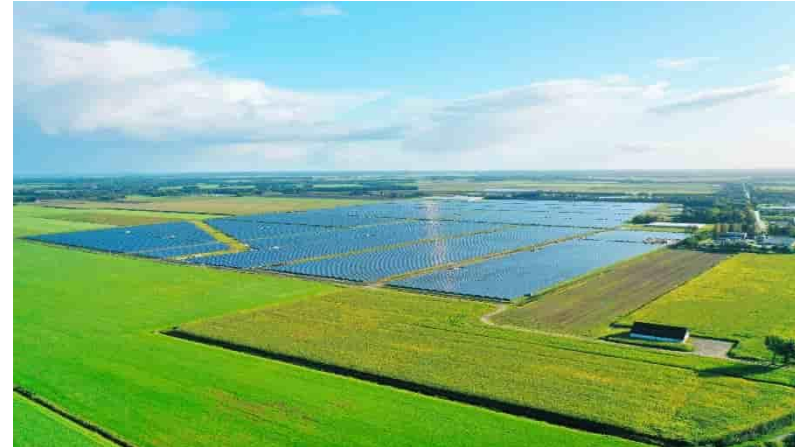
Midden-Groningen Solar Park, one of The Largest Power Stations in the Netherlands 103MW | The Netherlands
